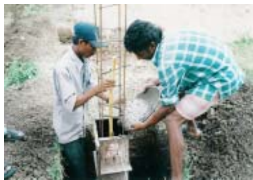
Workers add sand and mortar into the box molds for the wall pillars. This is very hard and intense work in India as you can see! They do not have the benefit of all the machinery that we have in the USA to build walls and buildings. Amazing!!
