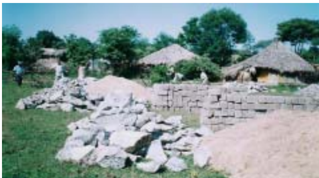
Above: The bricks, rock, sand and gravel that will construct the compound wall. Right: A 3-foot deep hole for securing one of the wall posts. It takes many of these to finish the wall.
