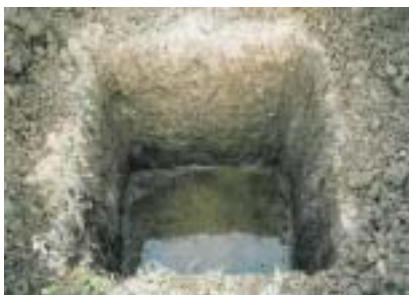
Above: The bricks, rock, sand and gravel that will construct the compound wall. Right: A 3-foot deep hole for securing one of the wall posts. It takes many of these to finish the wall.
