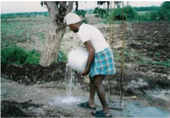
Above: Workers for Arms of Love Home for Children Below: Curing the foundation for the wall with water.
