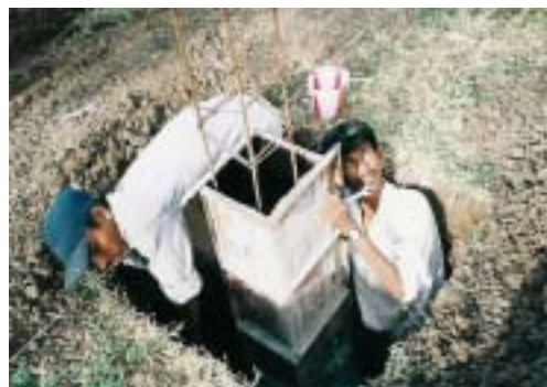
Workers add sand and mortar into the box molds for the wall pillars. This is very hard and intense work in India as you can see! They do not have the benefit of all the machinery that we have in the USA to build walls and buildings. Amazing!!
